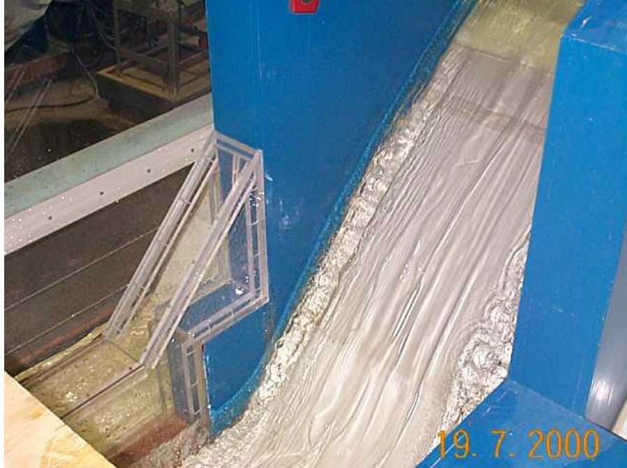
Photograph 13. RSW Alt 5, Flow Down Spillway Face
